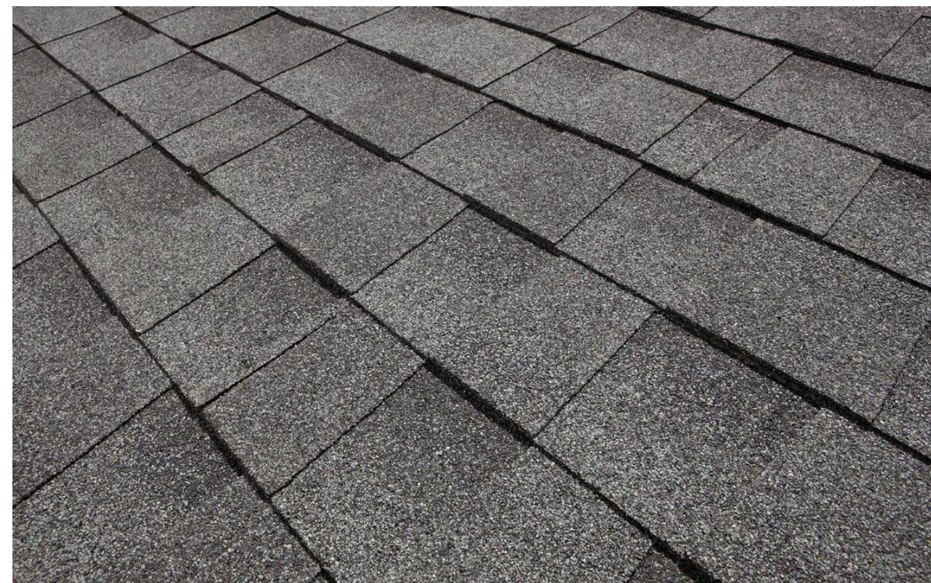
ASPHALT SHINGLE ROOFING (DARK GREY)
